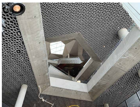
PYCA luminaires in the ceiling combs
