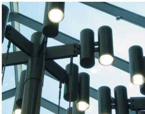
Spotlights in the tree structures
