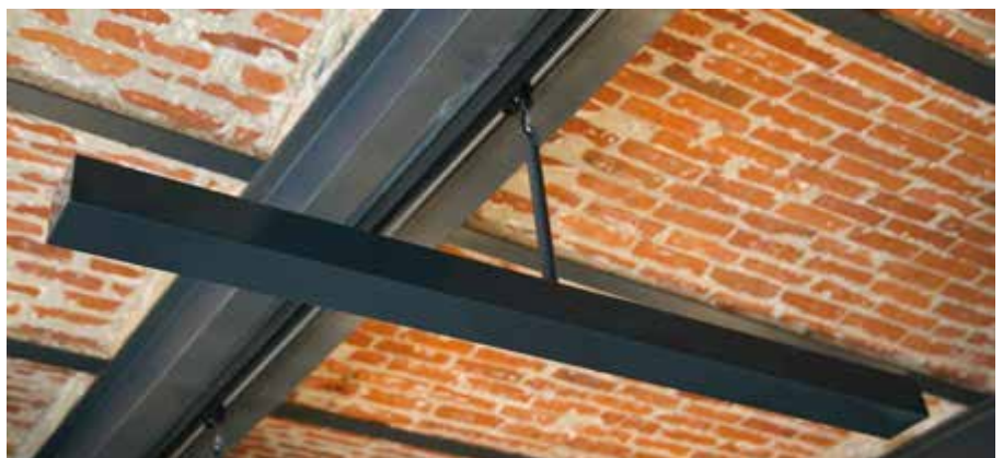
Indirect luminaire with track adapter
