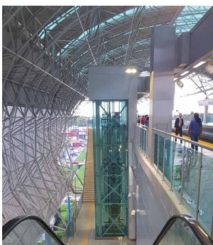
Elevator and column claddings
