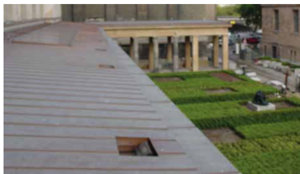
Facade floodlights in the colonnade roof
